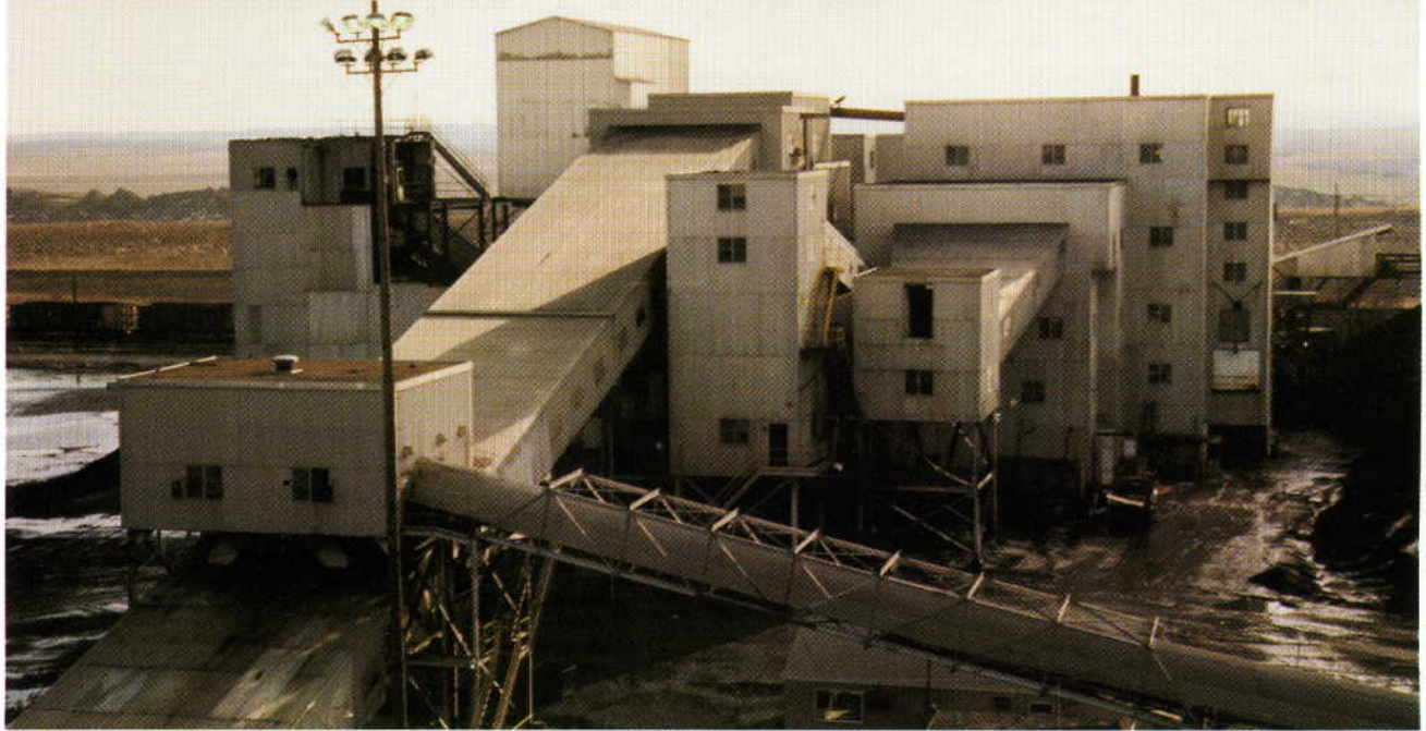
The $5 million fine coal plant addition to Arch of Illinois extends slightly above the preparation plant.
