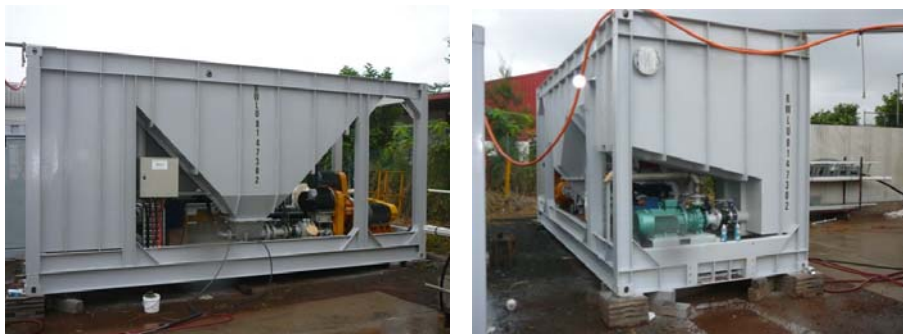
Figure 15 – Suspended sumps integrated into container module structure eliminating the need for structural bracing.
